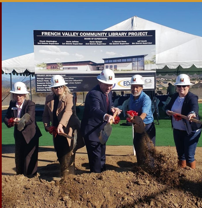
Supervisor Washington breaking ground at the site of the future French Valley library (1-10-20).
